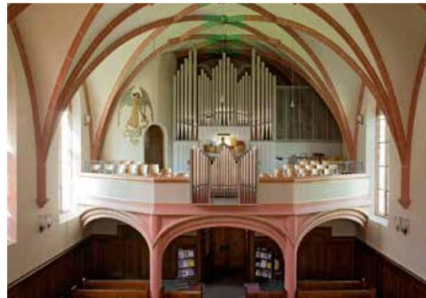
The brick-red cross-ribs are made of plaster and have no supporting function.
